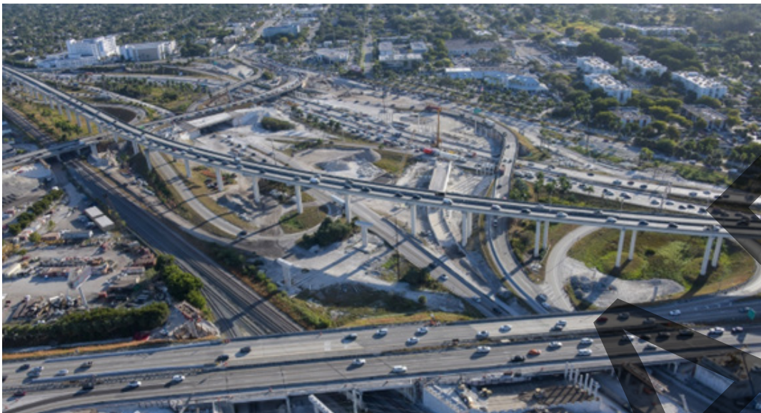
Northeast view through the core of the Golden Glades Interchange
